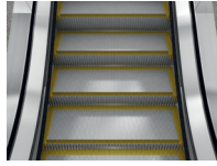
Plastic on sides and rear, and painted step nose
